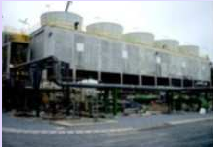
New Concrete Cooling Tower
