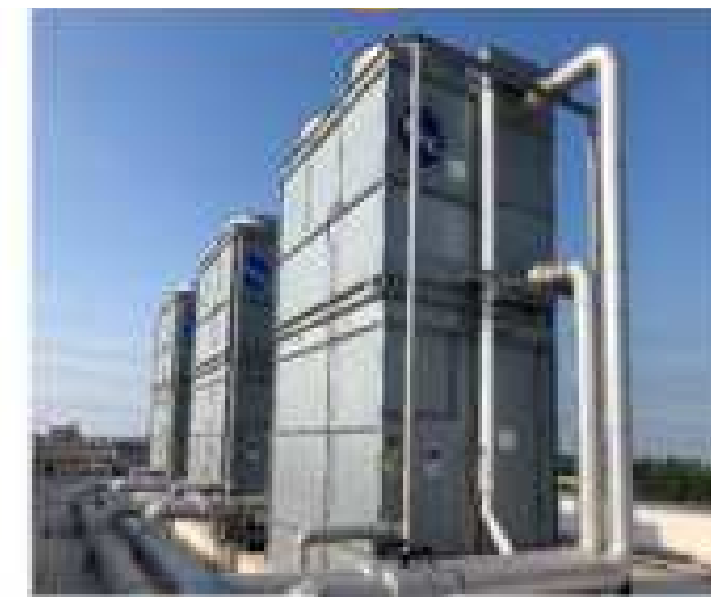
Evaporative Condenser
