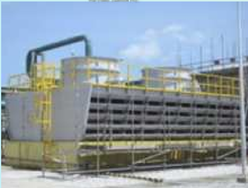
Reconstruction Cooling Tower
