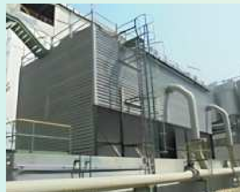
Reconstruction Cooling Tower
