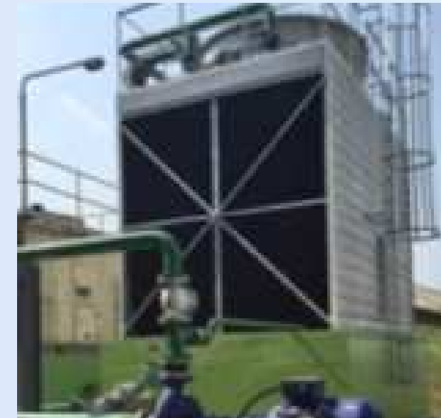
New Package Cooling Tower
